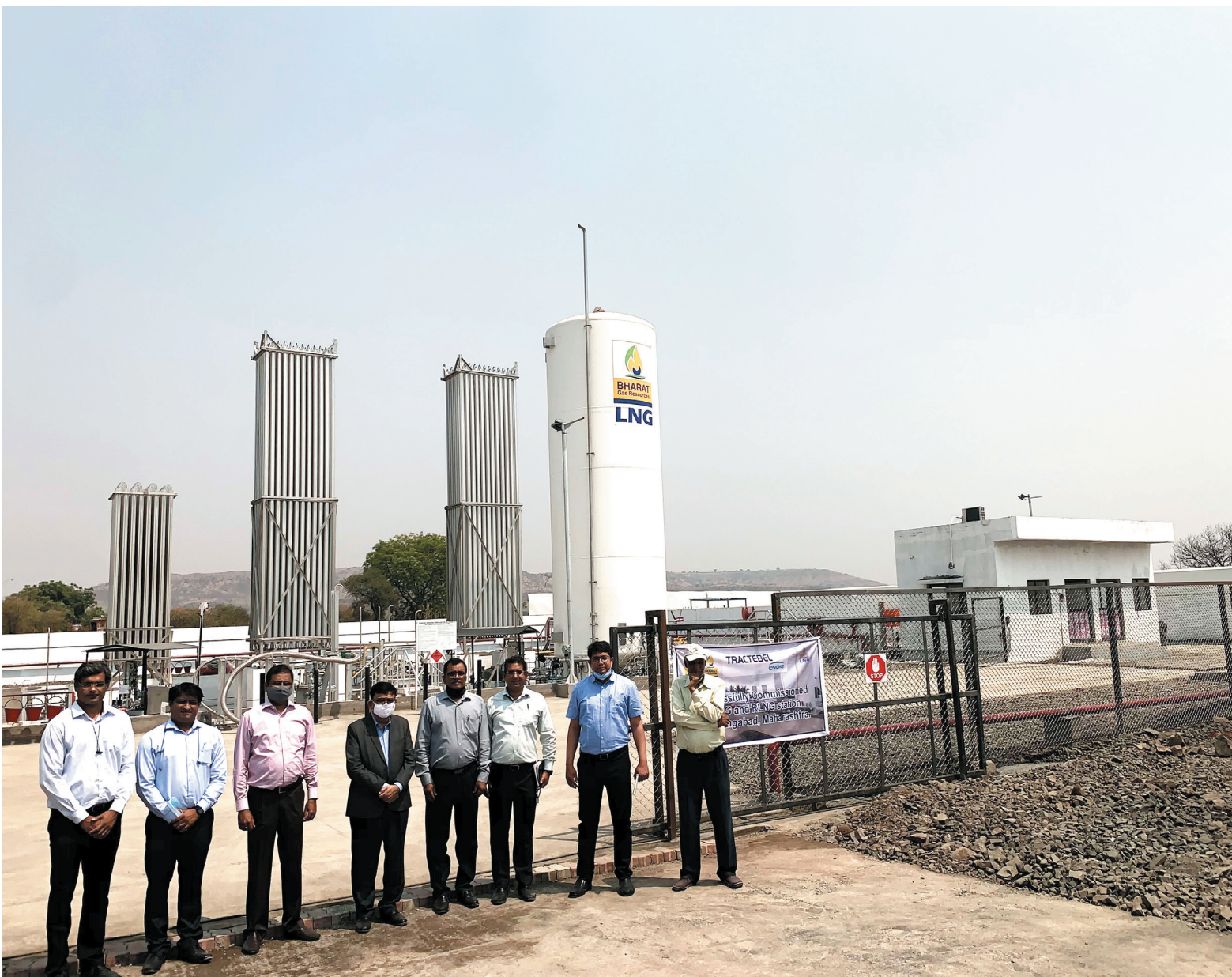
"Visit of Director at CGD Project site for overview of the project implementation"
